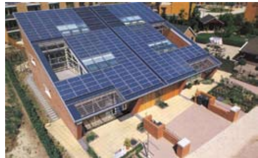
Figure 16: One of the experimental low energy houses in Nieuwland in Amersfoort, built in the early 1990s, demonstrated all kinds of techniques and systems Source: Wissing Town Planning and Urban Design
