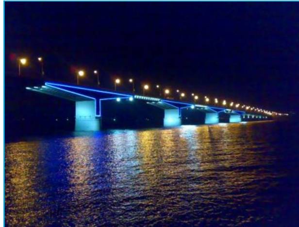
Bridge over River Kama in Perm
