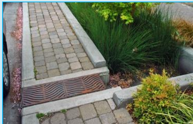
Green Street Bio-Swale
